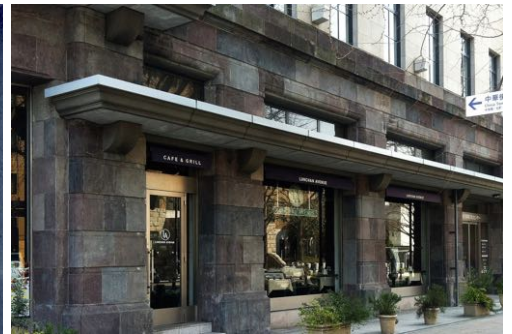
LA 2000 Yokohama Commercial Facility / Café+Grill
